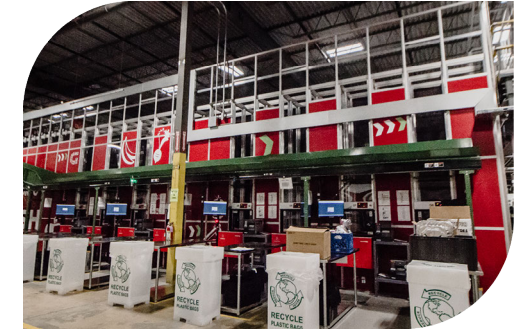
The GIANT Company opens state-of-the-art e-commerce fulfillment center.
